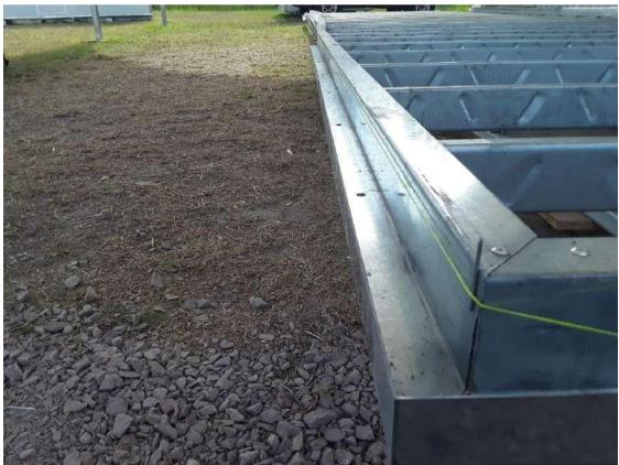
7 Paint corners, top edge and bottom holes of Z channel with With Rust Guard paint (similar to White Knight Rust Guard \*\* Not supplied by HC Containers)
