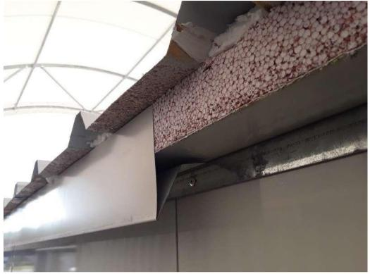
Silicone along both edges where drip line meets roof panel and roof cap.
