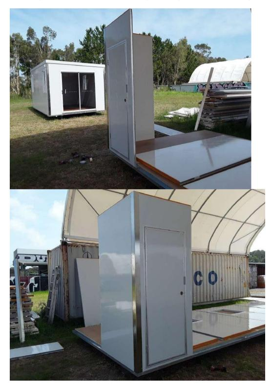
12 Continue standing wall panels, push them together until fitted tightly (no silicone or sealant required). Fit top-wall channel as you go along. Fit steel corners
