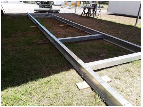
2 Measure diagonals to check the base is square. It may be necessary to use ratchet straps to pull the beams square. You may need to loosen the bolts connecting the beams in order to pull it square and straighten the beams - the bolts can be re-tightened after the flooring is screwed down
