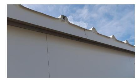
22 Cut internal corner flashing to length and rivet in place.
