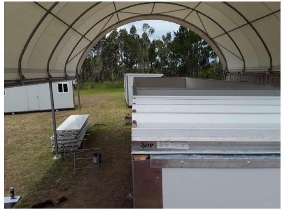
Panel should be flush with the front of the wall (long high side of building). Sight along the top of the roof sheet to ensure that the sheets do not run off line, adjust if needed and screw using 75mm Hex head screws in the valley of the high side to hold sheets in position until the flashings have been installed.
