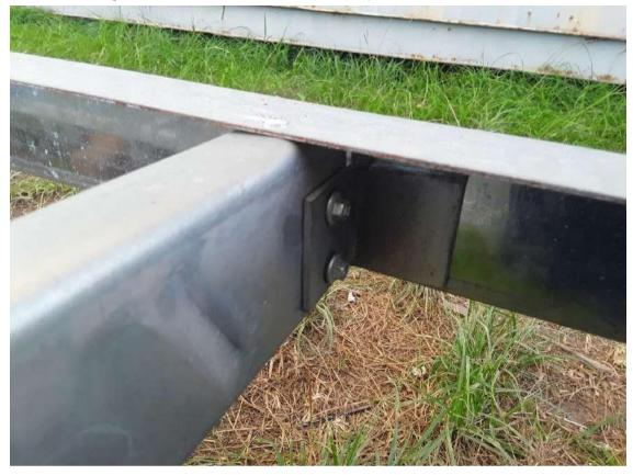
9 Mark the positions of the steel brackets and floor joists on the Z-channels (this will help with locating where to screw in later steps)
