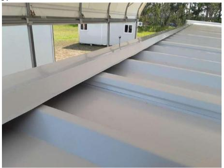
18 Fit and rivet the front and side eave covers. Front eave covers are secured by screwing into the peaks of the roof ribs through to the steel wall top channel. Silicone all joins.
