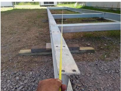
3 Bolt on the floor joists leaving the bolts loose. (first and last joists should have flat side facing out)
