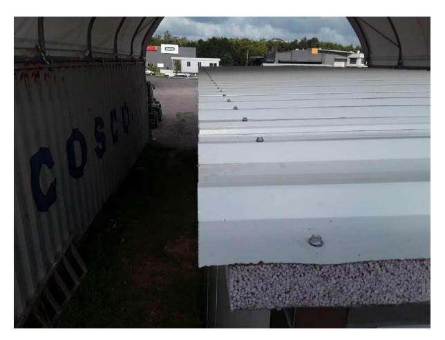
17 Temporarily fasten the front eave covers in position and mark the roof sheet ribs locations. Remove eave covers and cut out as marked so front eave covers fit snugly.
