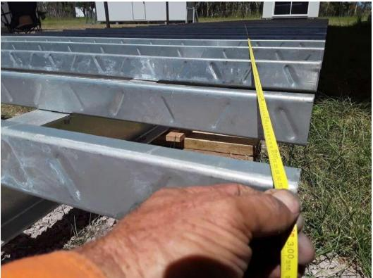
5 Rivet the Z-Chanels to joists at corners. Check diagonals for square. Adjust as necessary
