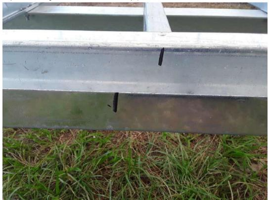
10 Position flooring boards and trim as necessary - The first board edge should land in the center of a floor joist (if it does not you need to start at the opposite side). Screw boards to joists, plane or sand joins. - some trimming of boards my be neccessary
