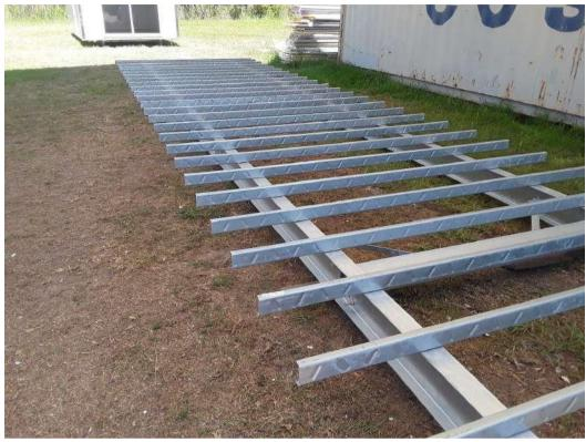
4 Tighten the end joists and check diagonals for square. Adjust as necessary. Tighten remaining joists - (Sight down the length of the building and get them as straight as possible)
