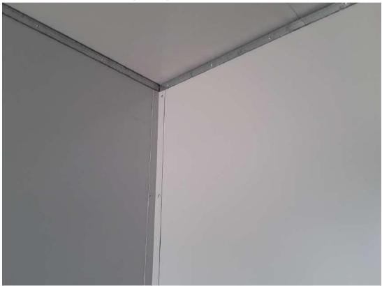
23 Peel the protective plastic on the internal and external walls and internal ceiling - Use a Stanley knife to score along top and bottom and peel.
