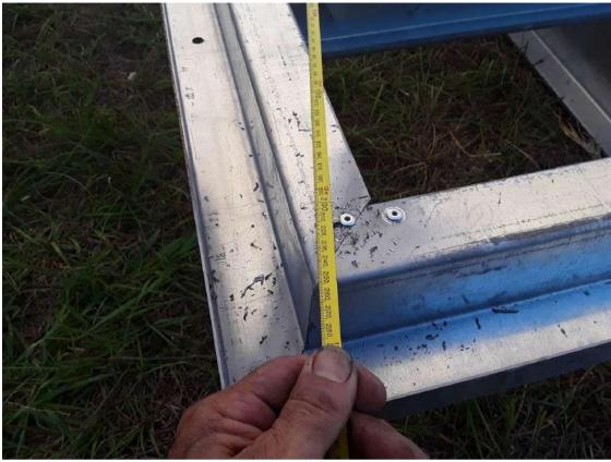
6 Run a string line along the Z-channels and rivet the channels at the end of each floor joist
