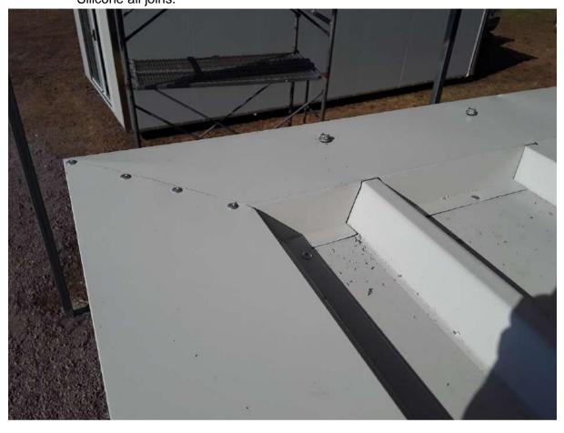
19 Push the rear drip line flashing between the top of the roof sheet and the polystyrene (using a knife or paint scraper to loosen the polystyrene first can help) then rivet in place.
